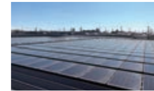
Solar panel installation
