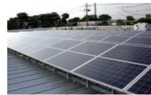
Solar panel installation
