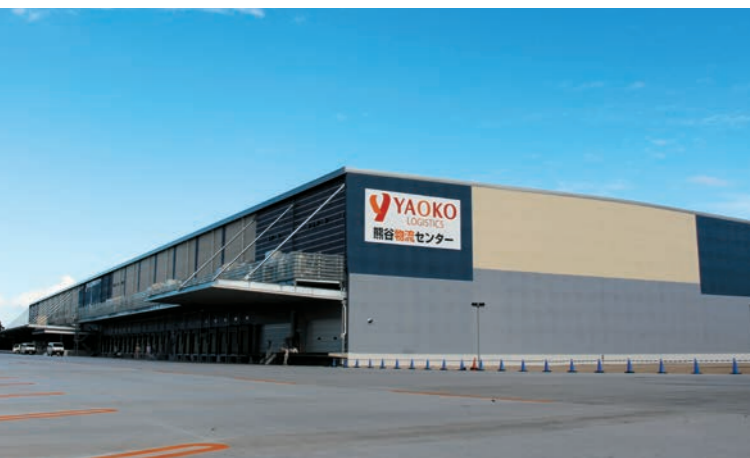
<Kumagaya Distribution Center>
